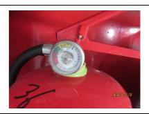
No.27 Fire extinguisher with proper pressure
